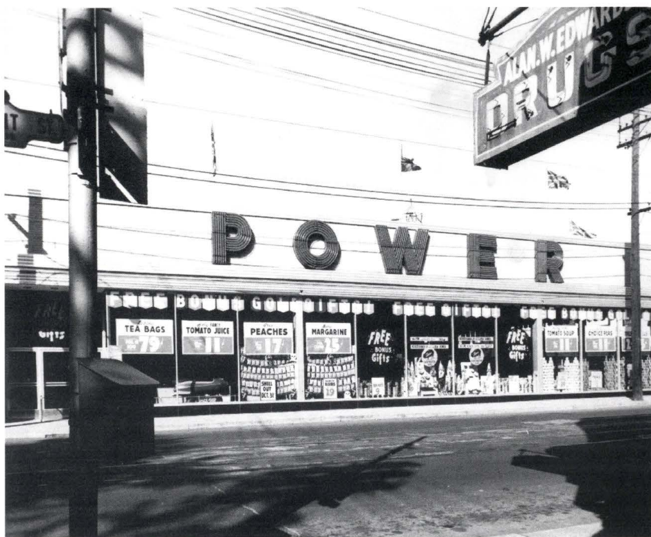
The glass-fronted Power supermarket (now Loblaws) at Huron and Dupont, circa 1958.
